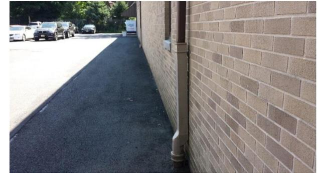
Parking spaces can be repaved with porous asphalt to infiltrate parking lot runoff. A bioretention system can also be installed in the turf grass area off of the southeast corner of the CYO building, where water currently pools. This rain garden could also infiltrate runoff from the adjacent Metuchen Municipal Court. A preliminary soil assessment suggests that the soils have suitable drainage characteristics for green infrastructure.
