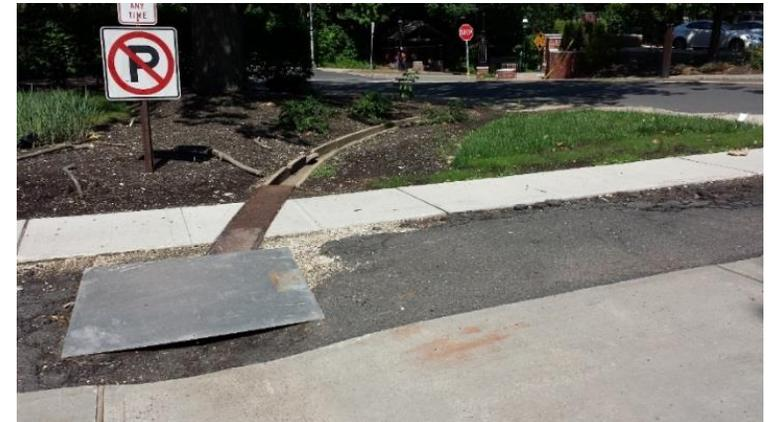
The Post Office parking lot is in poor condition and ponding occurs after rain events. Parking spaces can be replaced with pervious pavement to reduce impervious cover and promote infiltration. The concrete flow channel near the employee driveway can also be replaced with a bioswale to remove pollutants and allow stormwater to infiltrate. A preliminary soil assessment suggests that the soils have suitable drainage characteristics for green infrastructure.
