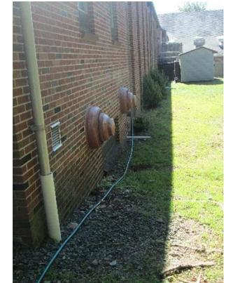
The church sits on a hill and runoff from the pathway and the downspouts is causing erosion and gulying. A bioretention system can be installed to help manage stormwater in this area. Rows of parking spaces can also be converted into pervious pavement to infiltrate parking lot runoff. A preliminary soil assessment suggests that the soils have suitable drainage characteristics for green infrastructure.
