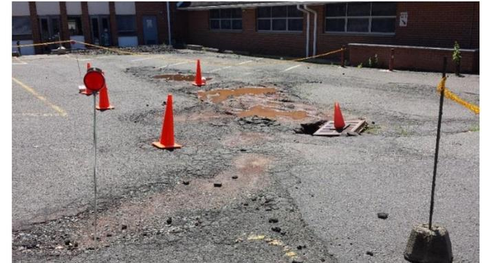
This church has severe damage to its northern parking lot near the building. This area can be replaced with pervious pavement to infiltrate parking lot runoff. Bioretention systems can also be installed to capture, treat, and infiltrate additional parking lot runoff as well as roof runoff. A preliminary soil assessment suggests that more soil testing would be required before determining the soil's suitability for green infrastructure.
