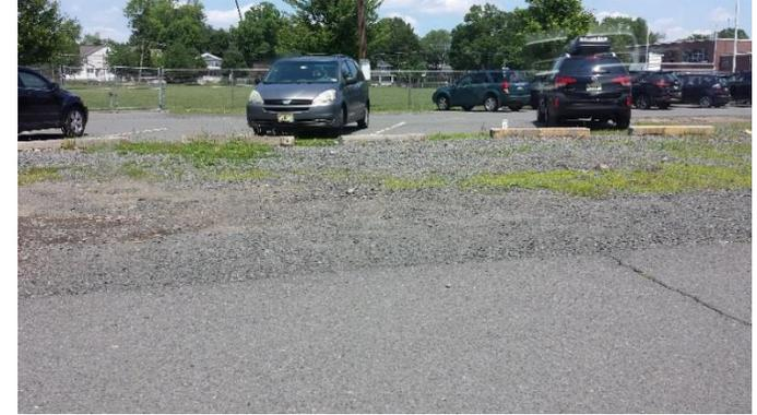
The parking lot is in poor condition. Rows of parking spaces can be replaced using pervious pavement to promote infiltration. A preliminary soil assessment suggests that the soils have suitable drainage characteristics for green infrastructure.
